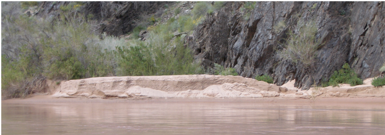
Figure 1. Coulomb-type slope failure.
