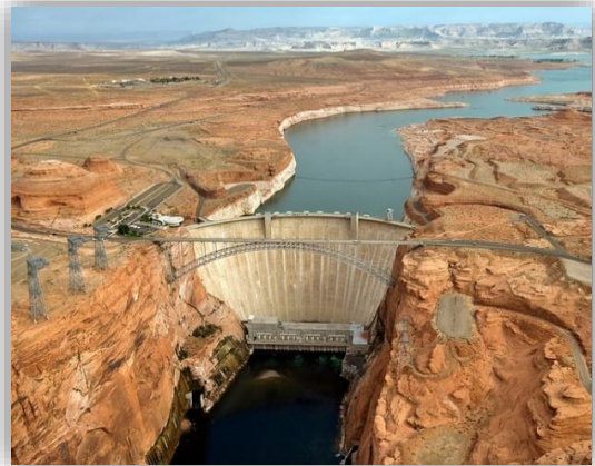
Photo: Glen Canyon Dam
