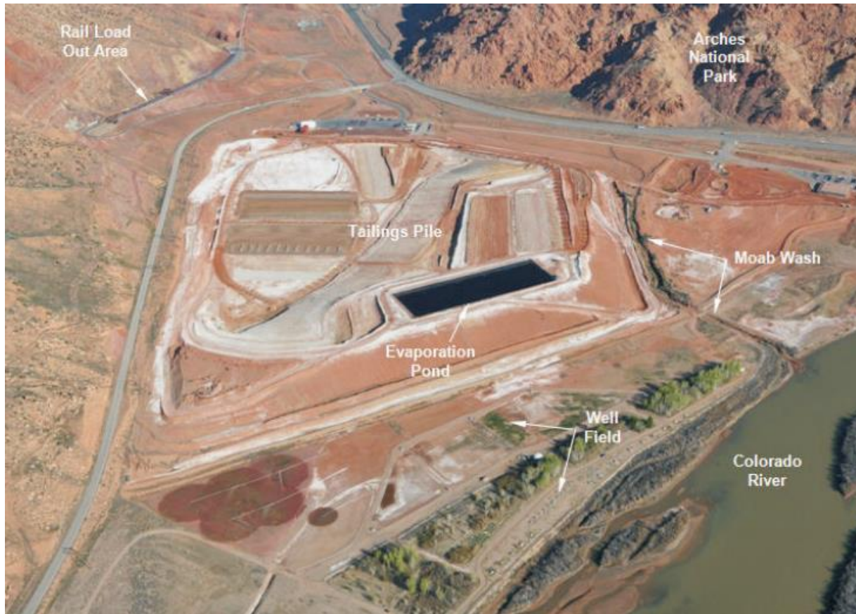
Fig. 4: Aerial view of the Moab Mill tailings pile and well field (USDOE, 2015)
