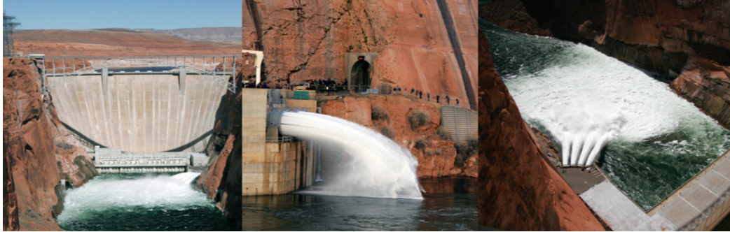
Figure 3 Images of the Glen Canyon Dam releasing water through bypass tubes. Images from the US Bureau of Reclamation 2019.
